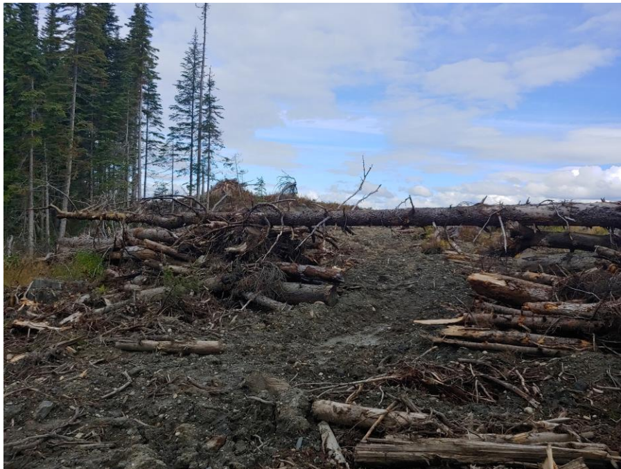
Figure 4. Picture of completed CWD corridor that provides connectivity across rehabilitated road located within the road right-of-way between Cutblocks A-3 and A-4.
