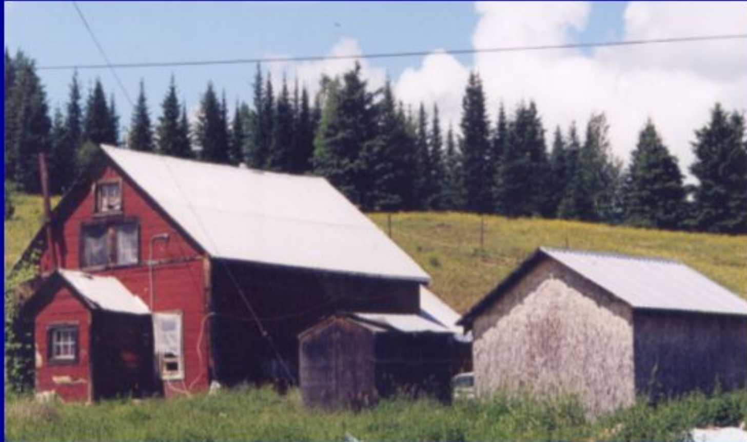
Ego Bjorklund's log house, covered over with red roofing paper. Aleza Lake
