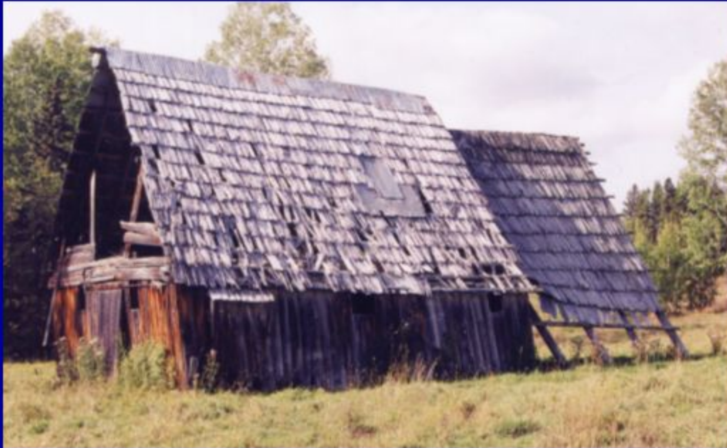
Bearman shake-roofed barn. Newlands
