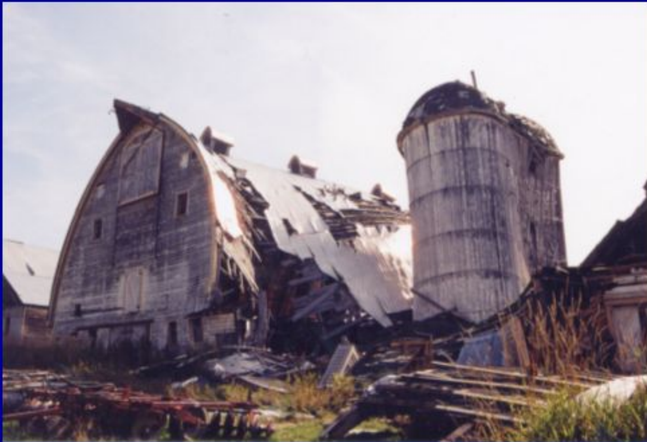
The old dairy remains at Giscome
