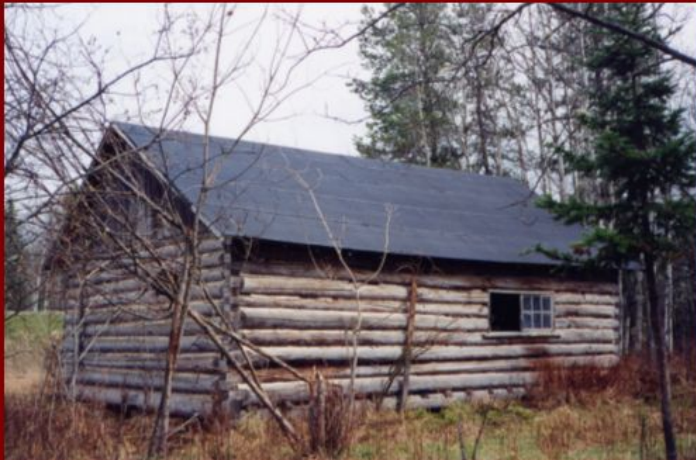
The Hixon seed-cleaning plant across from Baehrs
