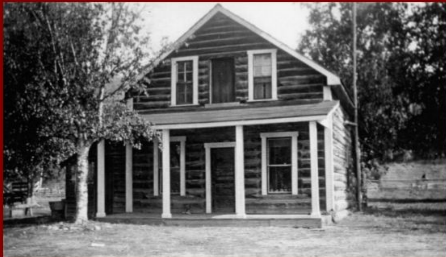
The Dale log house built circa 1918-20
