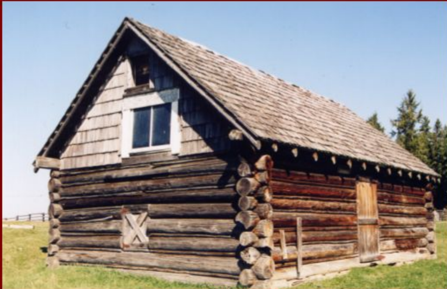
Log barn at Kolling Road
