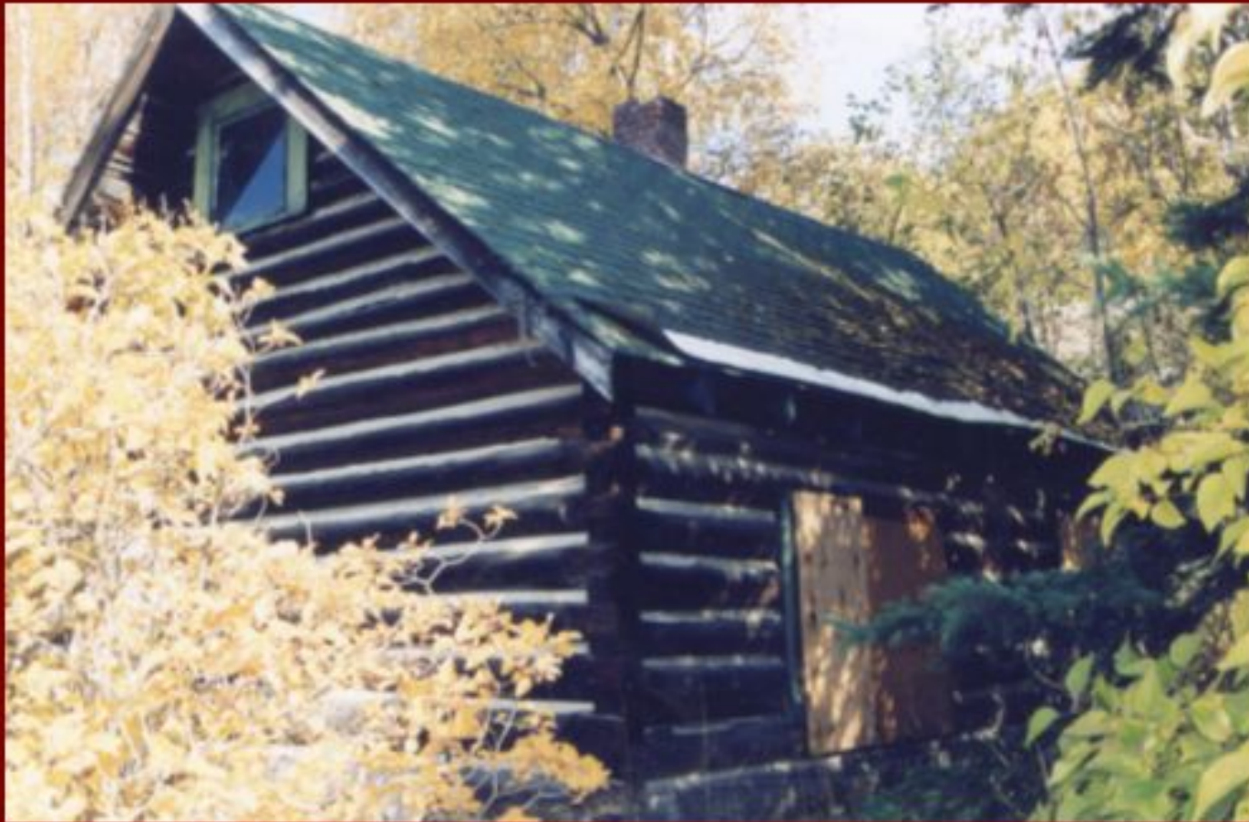
The Bell house on Woodpecker Landing Road
