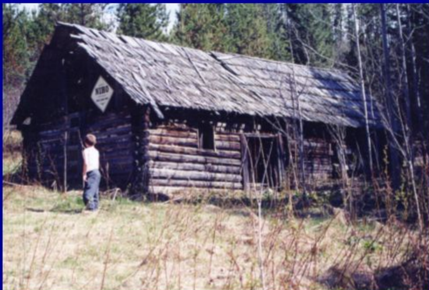
Miskoski barn on Patterson Road
