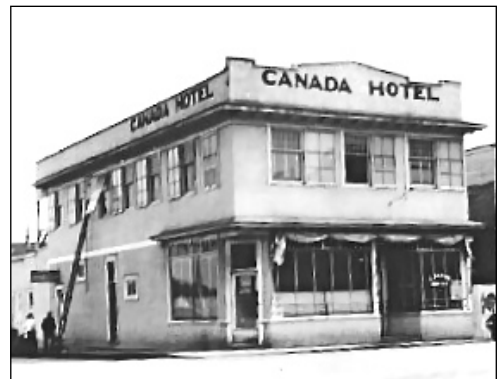
The Canada Hotel (ca. 1930) was typical of small, working-class hotels. The Canada was demolished in 1991 for the courthouse.
