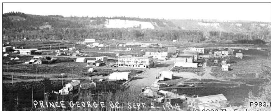
King George Hotel ( centre of photo) under construction on George St. Photo: Exploration Place
