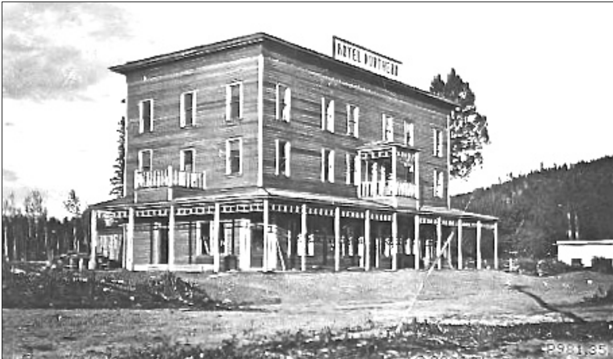
The second Hotel Northern built 1911. This is the first stage of construction. Note the pattern of window placements on the front facade.
