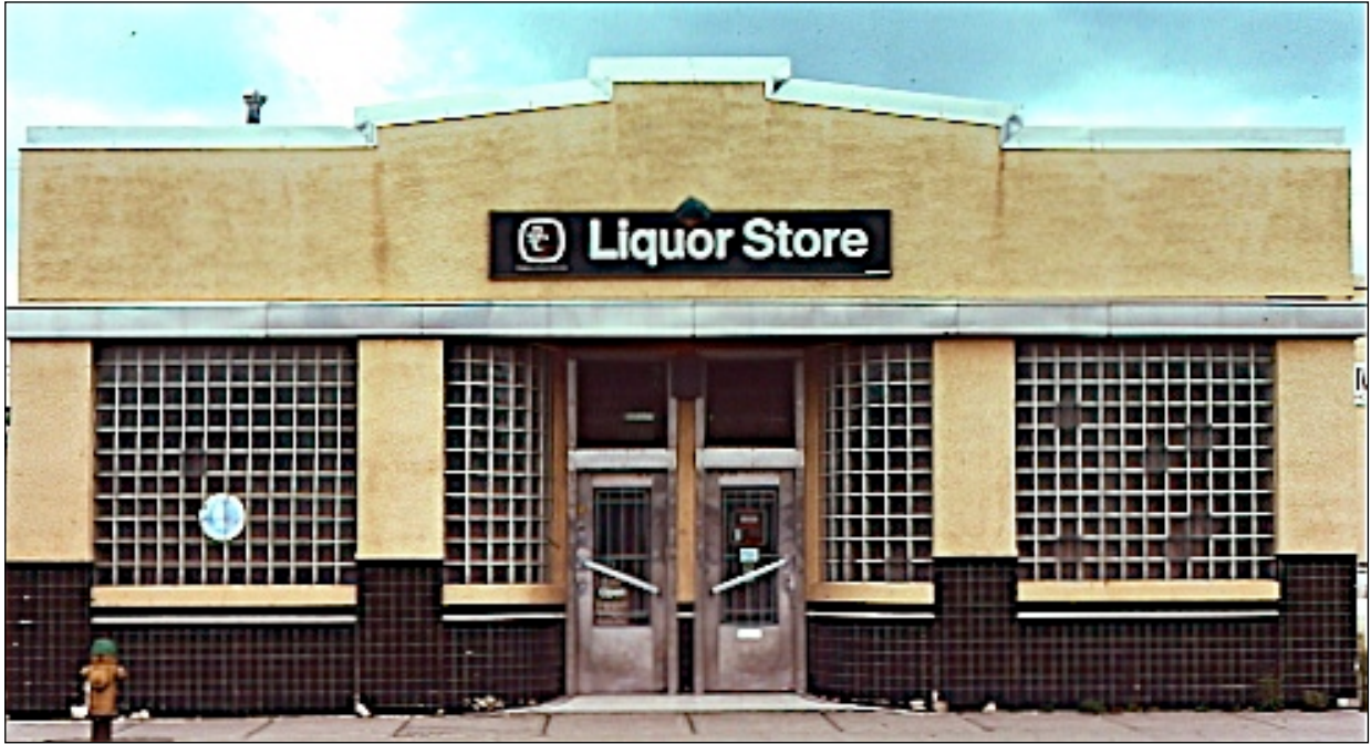
Front facade with details of glass block windows and stainless steel doors. Photos: K. Sedgwick
