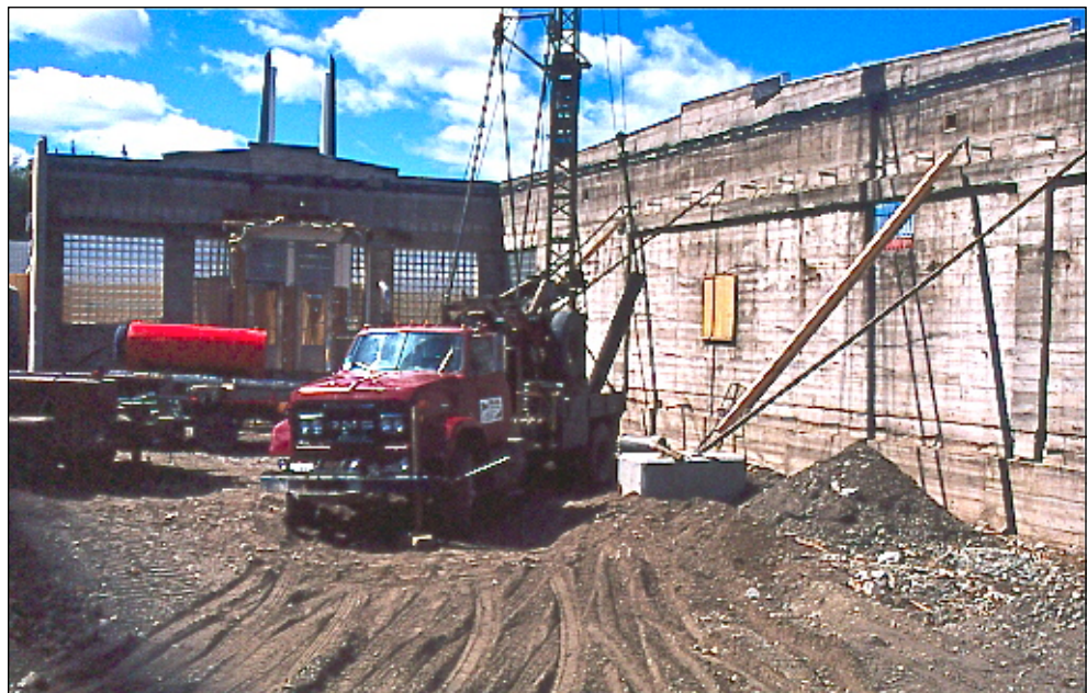
The designated front wall, with glass block windows, and side wall were retained as the rest of the building was demolished.
