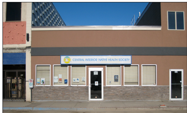
"Modern" facade in 2011 on what may be Anderson's 1937 liquor store. Photo: K. Sedgwick
