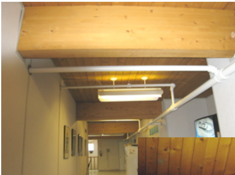
three laminated spruce beams in hallway
