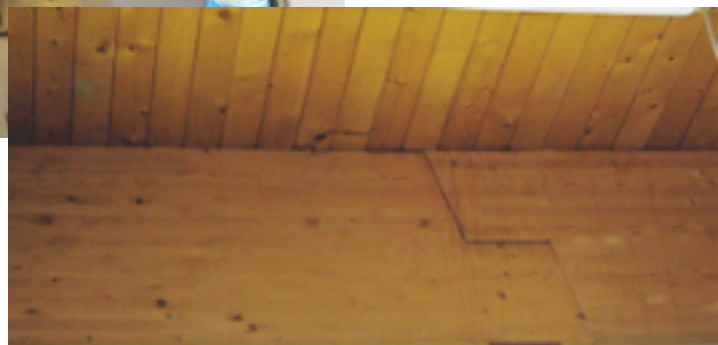
detail of join in spruce beam
